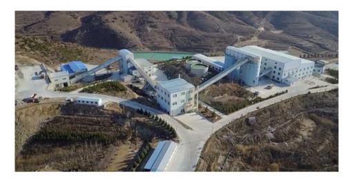
Our integrated ore processing facility comprises one mill to process the ores mined from our Songjiagou Open-Pit Mine and Songjiagou Underground Mine. Our ore processing plant has a total surface area of approximately 0.9 ha. The total designed ore processing capacity of our ore processing facility amounted to approximately 2,000 ktpa (or 6.0 ktpd) as at 30 June 2023.
