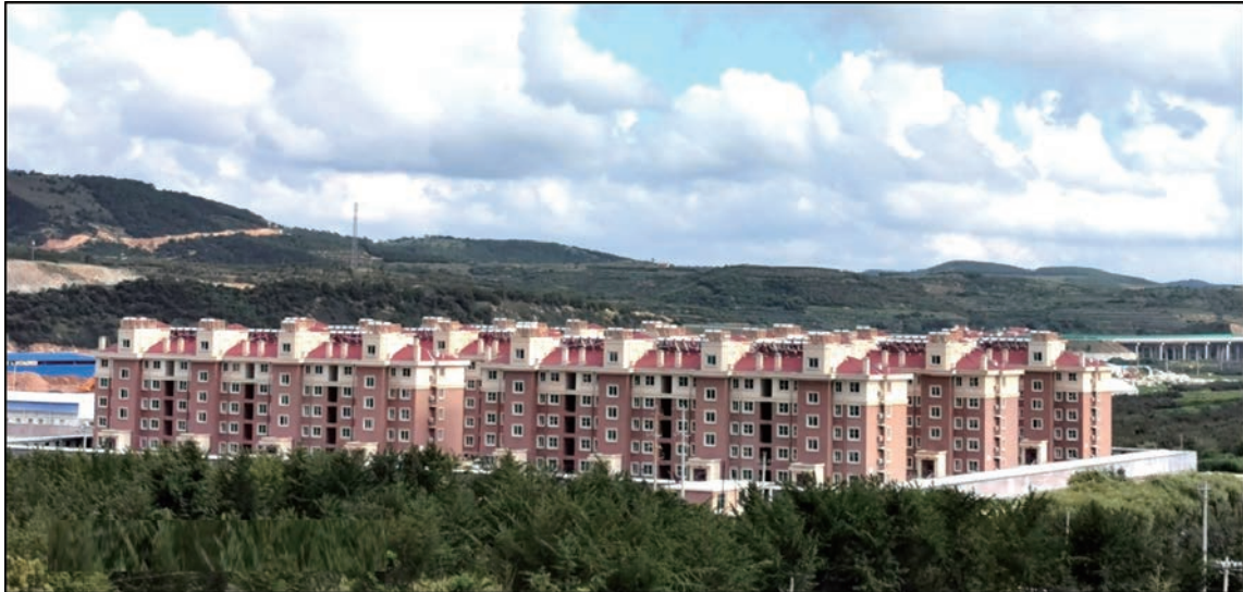
Figure 3-1: Typical Resident Apartments
