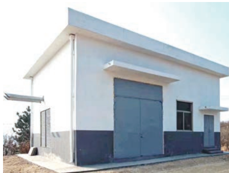
room for diesel generator
