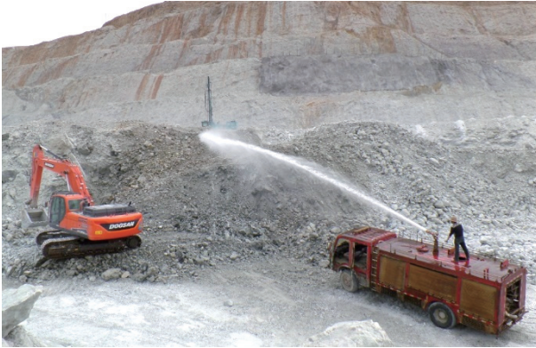
Figure 18-1: On-site Water Sprinkling
