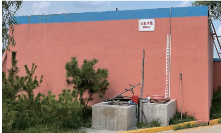
Figure 14-9: Elevated Water Tank
