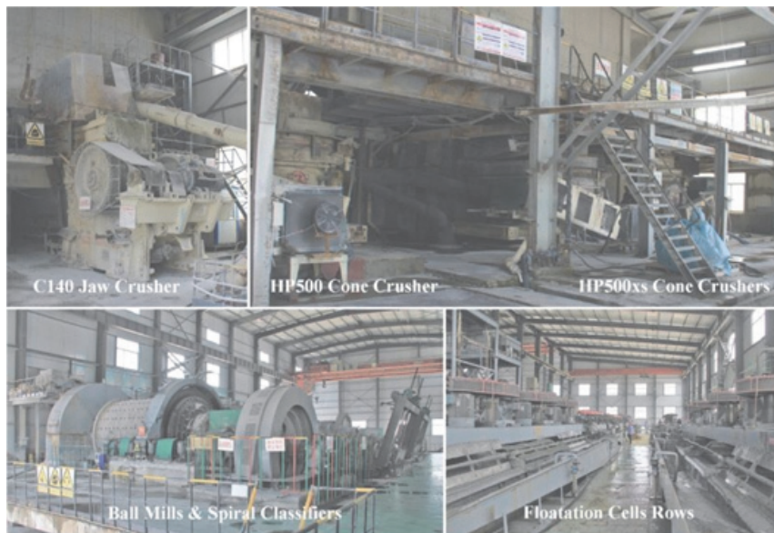
Figure 15-6: Photos of Processing Equipment
