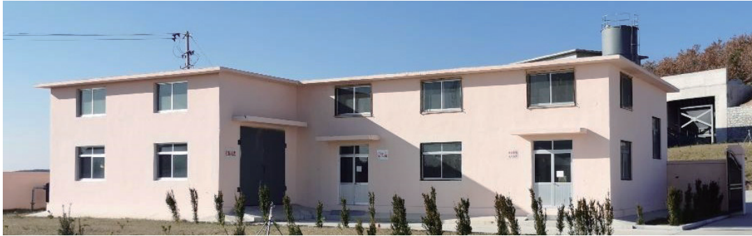
building for compressed air and power distribution
