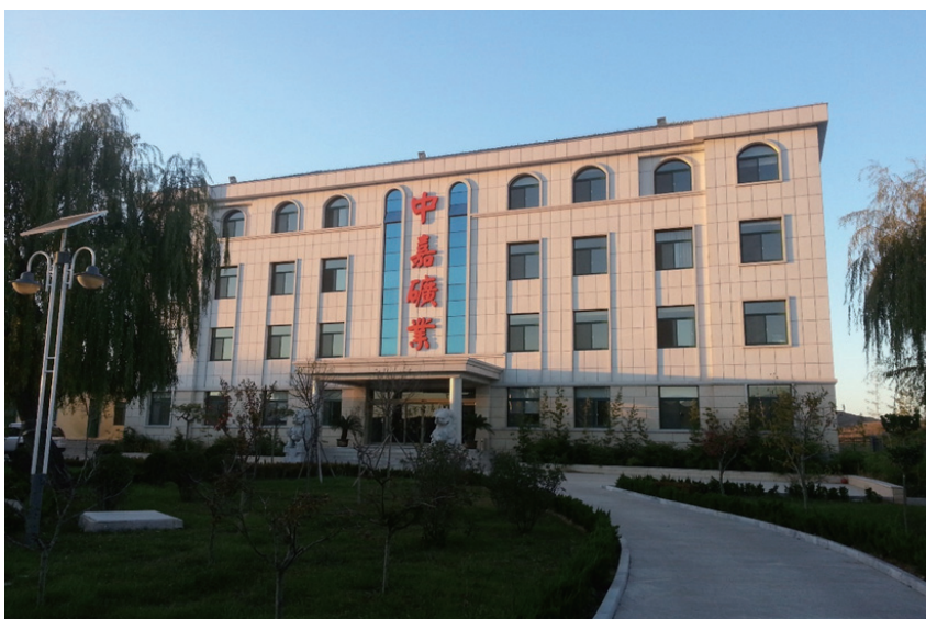
Figure 16-6: Off-site Office Building
