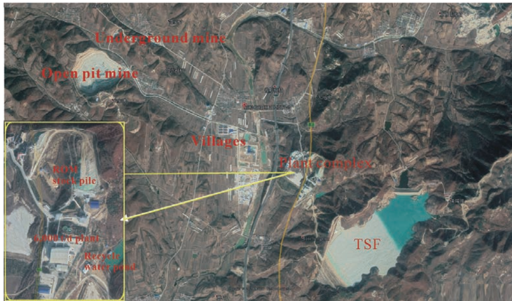
Figure 15-1: The Location of Mining and Processing Facilities
