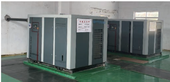
single screw air compressor
