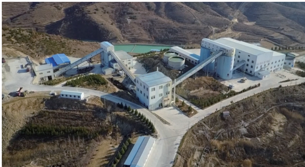
Figure 15-2: Aerial Photo of the Processing Plant
