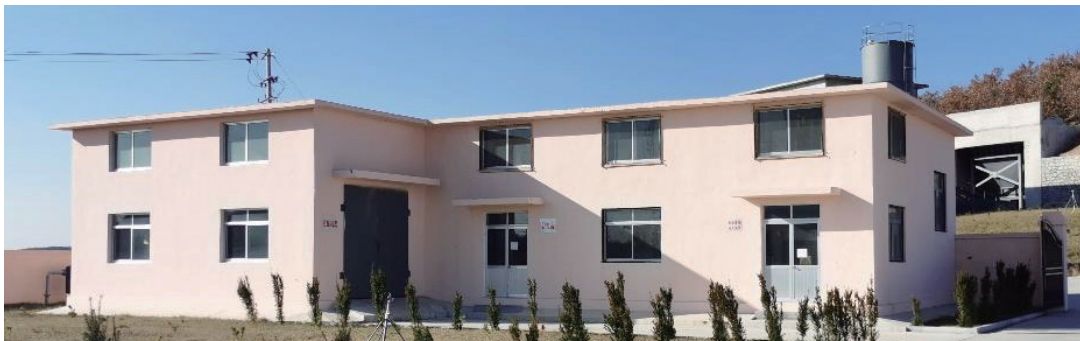
壓縮空氣及配電樓
