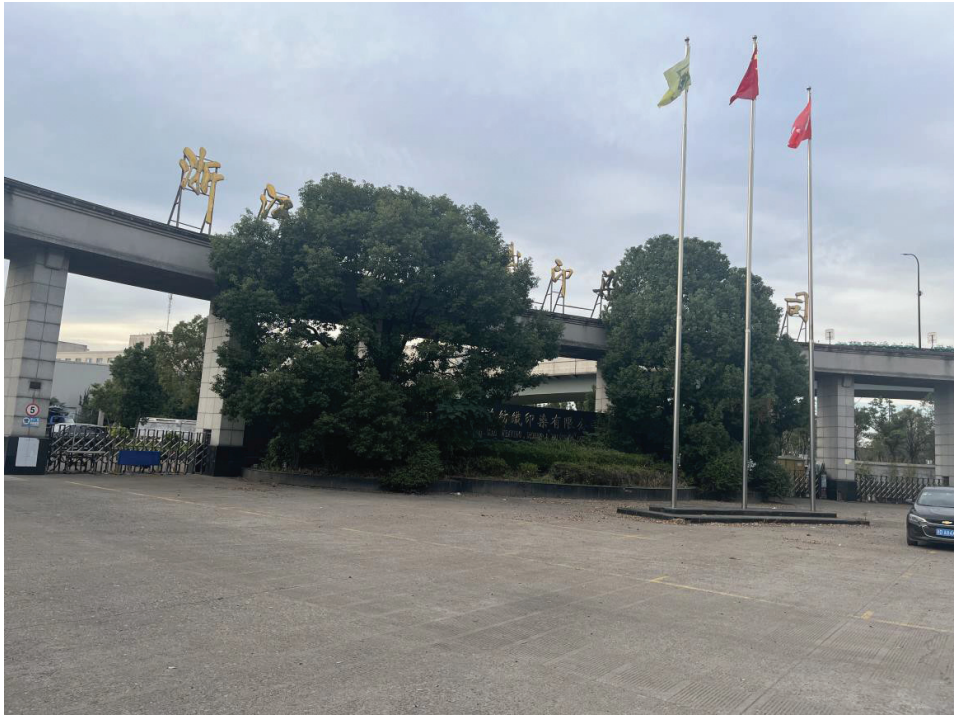
Appendix II Photos Related to On-site Survey of the Valuation Object
