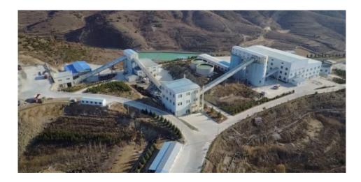
Our integrated ore processing facility comprises one mill to process the ores mined from our Songjiagou Open-Pit Mine and Songjiagou Underground Mine. Our ore processing plant has a total surface area of approximately 0.9 ha. The total designed ore processing capacity of our ore processing facilities amounted to approximately 2,000 ktpa (or 6.0 ktpd) as at 30 June 2023.
