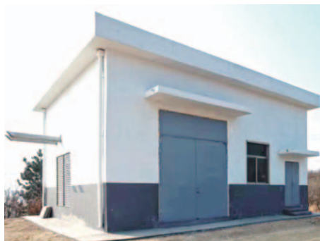
room for diesel generator
