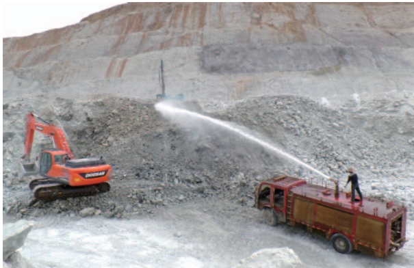
Figure 18-1: On-site Water Sprinkling
