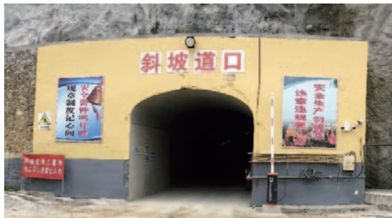
Access ramp's portal
