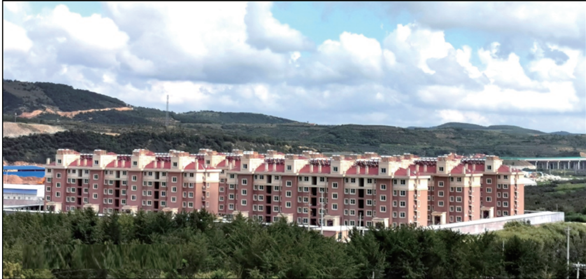
Figure 3-1: Typical Resident Apartments
