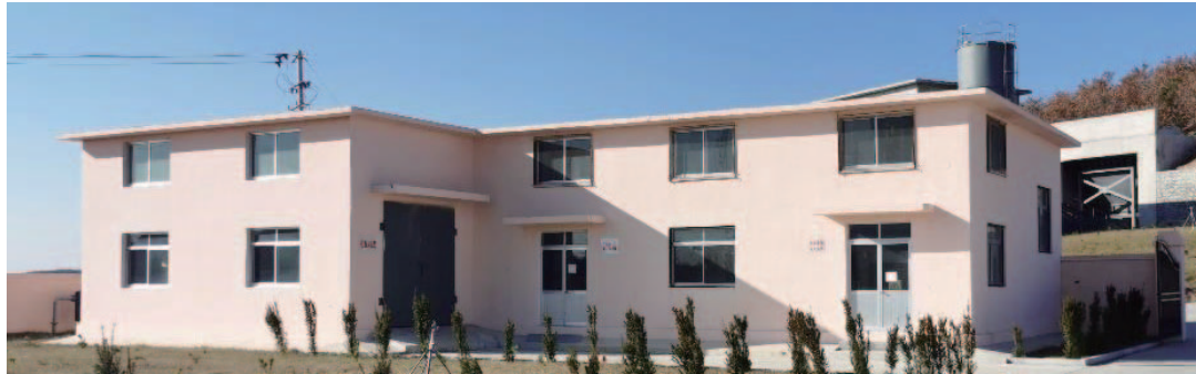
building for compressed air and power distribution
