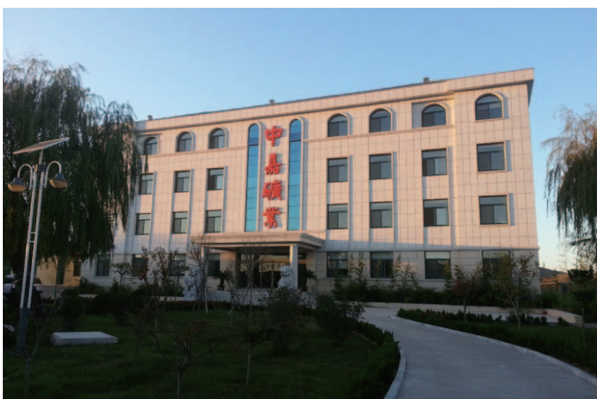
Figure 16-6: Off-site Office Building
