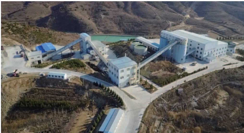
Figure 15-2: Aerial Photo of the Processing Plant
