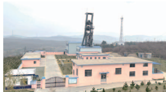
Industrial site of auxiliary shaft
