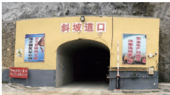
Access ramp's portal
