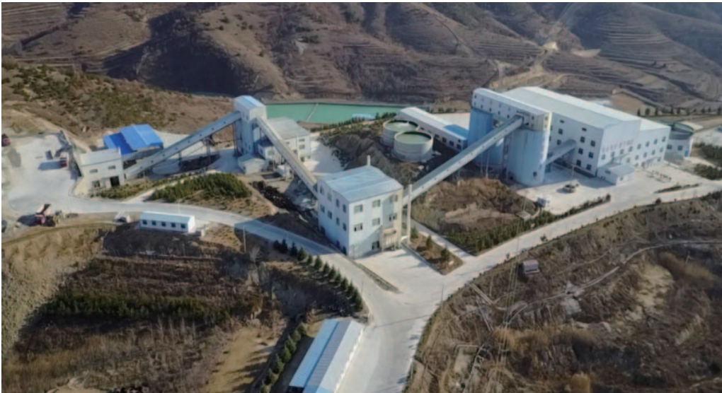
Figure 15-2: Aerial Photo of the Processing Plant
