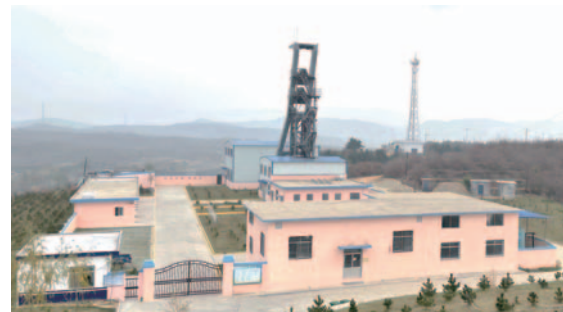
Industrial site of auxiliary shaft
