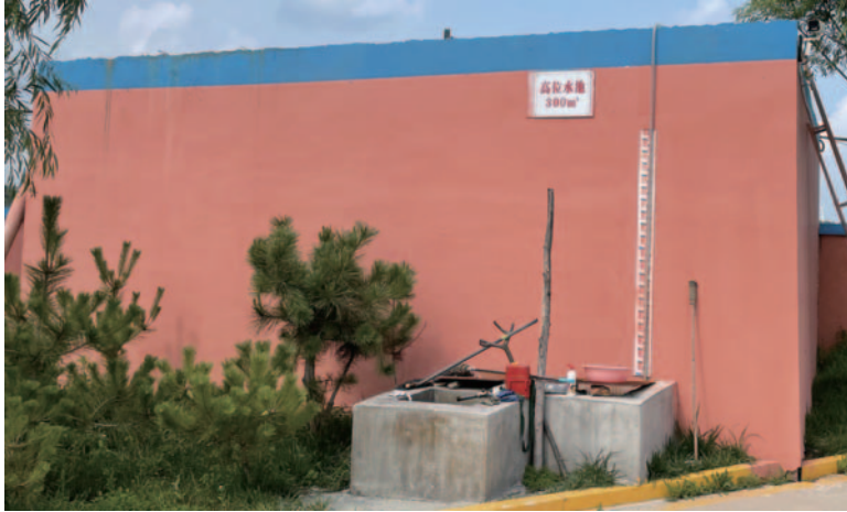
Figure 14-9: Elevated Water Tank
