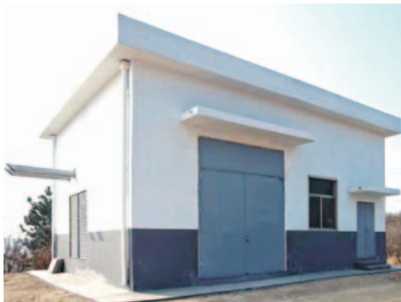
room for diesel generator
