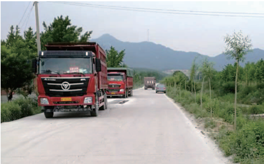
Figure 16-1: Concrete Paved Road Connecting Mining Area and Processing Plant
