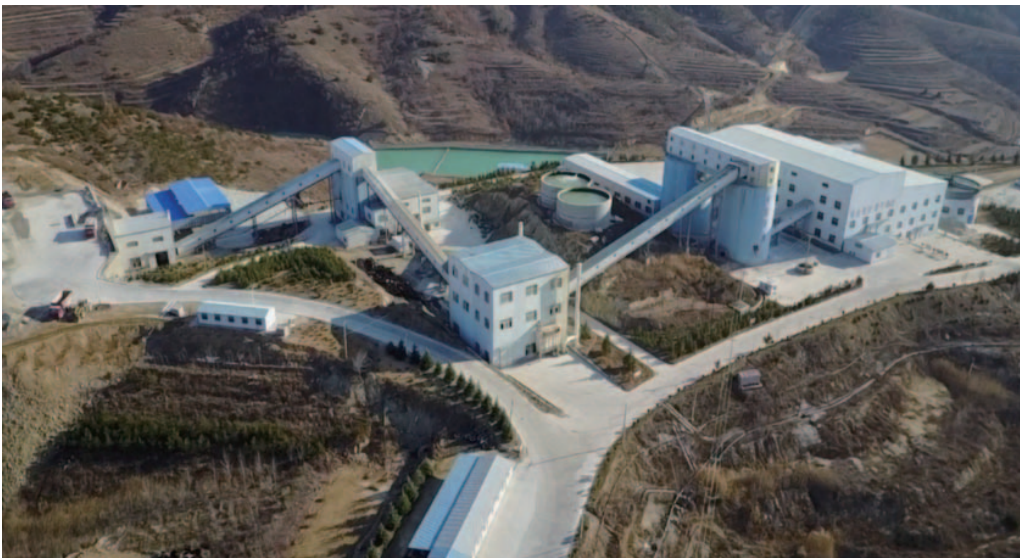
Figure 15-2: Aerial Photo of the Processing Plant
