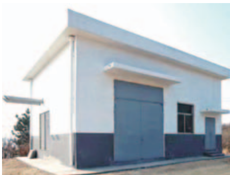
room for diesel generator
