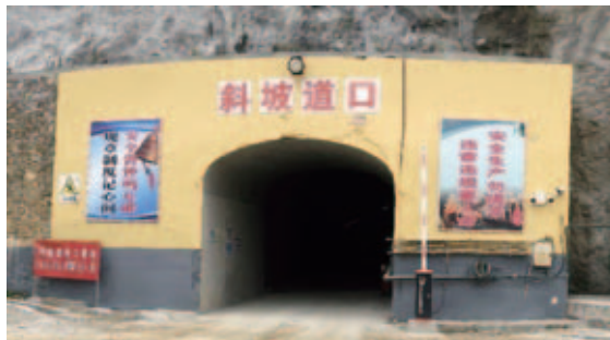
Access ramp's portal
