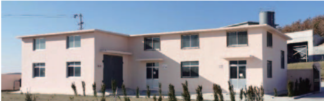
building for compressed air and power distribution
