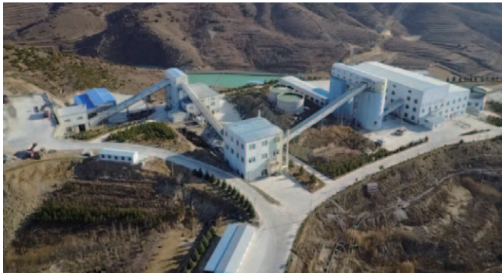
Figure 15-2: Aerial Photo of the Processing Plant
