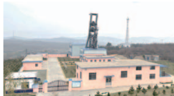
Industrial site of auxiliary shaft
