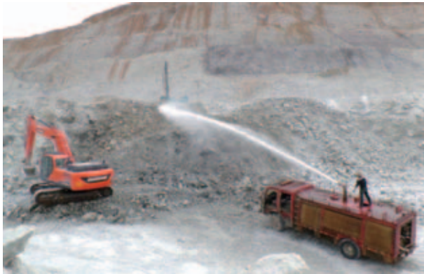
Figure 18-1: On-site Water Sprinkling
