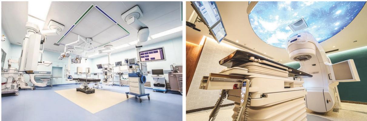
Digital integrated class 100 laminar flow operating room and linear accelerator in Guangzhou Hospital
