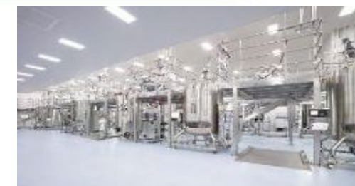
MFG8 in Hebei Digital platform for energy optimization
