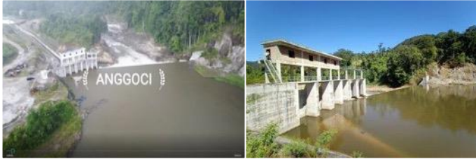
ANGGOCI 10MW Commercialised since 15 June 2023
