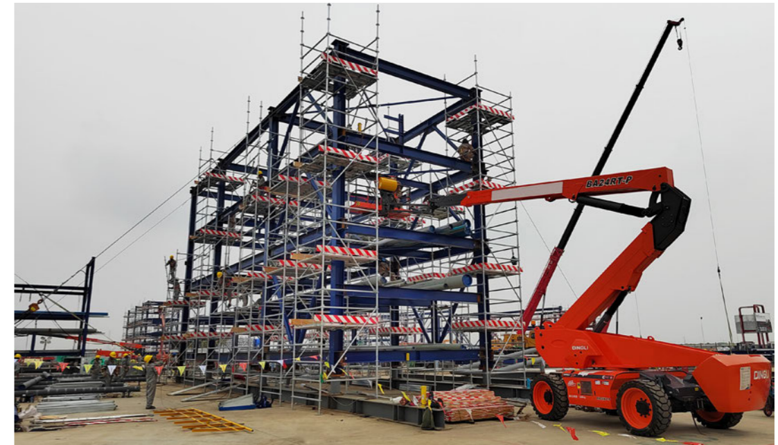
South Port Ethylene Process Corridor Module Construction
