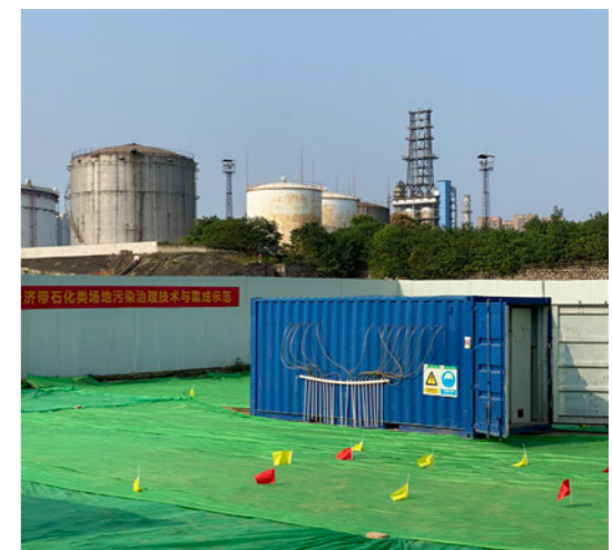
Green Remediation Technology and Equipment System at the Sino-Korean (Wuhan) Petrochemical Demonstration Site
