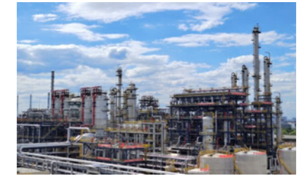
CHP Process Epichlorohydrin Unit
