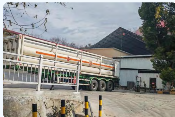
Hydrogen-blended Combustion Experiment Project of Digang Conch
