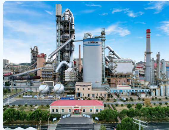
CCUS Project of Baimashan Cement Plant
