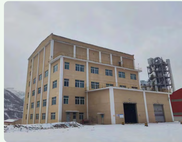
Collaborative Treatment of Cement Kilns of Linxia Conch
