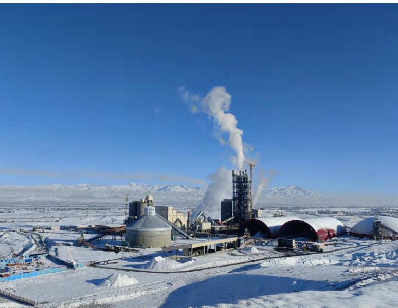
Tashkent project was completed and put into operation
