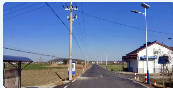
Pingding Village Illumination Project
