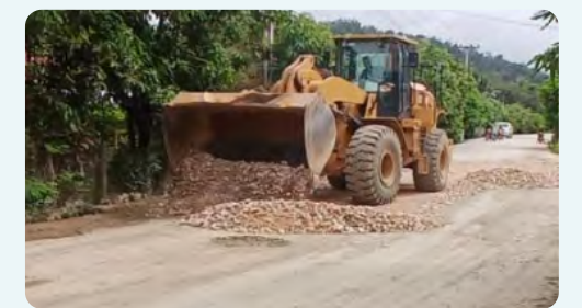
Laos Luang Prabang Conch Cement Repairs Public Road
