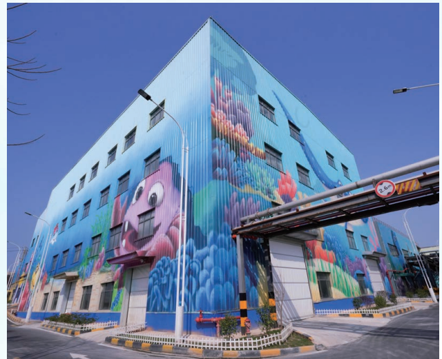
The Environmental Company Nanning Bioland Organic Waste Treatment Project
