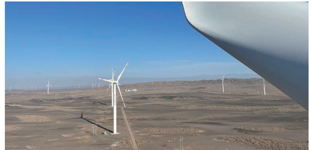
Qianxin Wind Power Plant in Xinjiang
