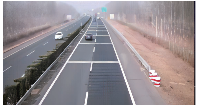
Active Traffic Control
