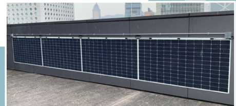
33 Des Voeux Road Central in Hong Kong
