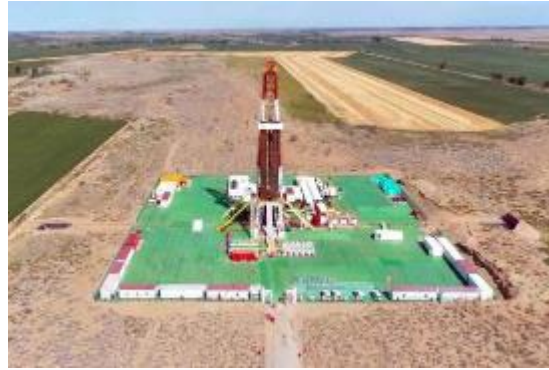
▲ Laying dust-proof nets at construction sites
