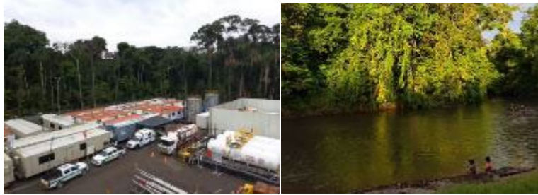
▲ Working site of Ecuadorian project
