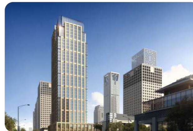
Guangzhou NCI Building
