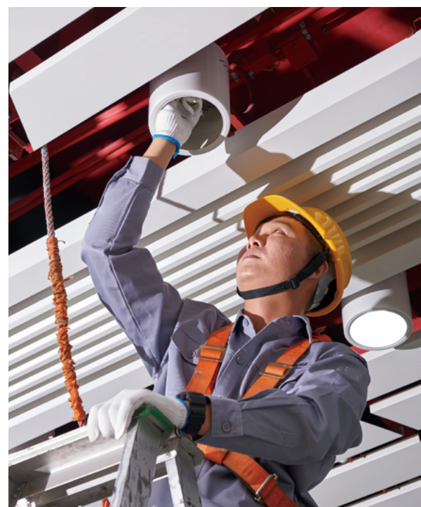
Installation of Energy-saving Lamps in Basement
