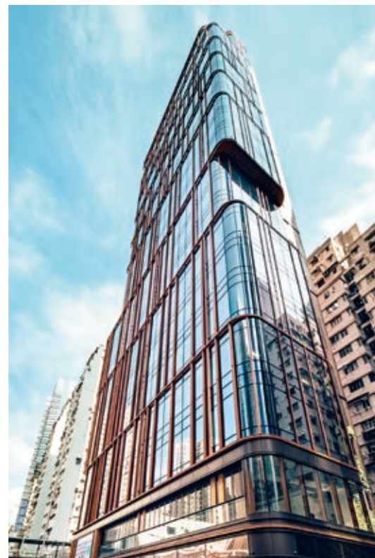
Newly added to our office portfolio in 2023, 228 Electric Road provides exquisitely designed offices in the vibrant heart of the North Point business district
