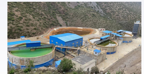
Jiama Mine Sibugou Water Treatment
