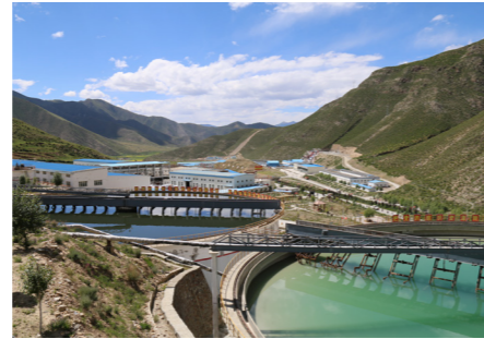
Jiama Mine adopted the flotation wastewater reusing and treatment technology to achieve "zero discharge" of sewage
