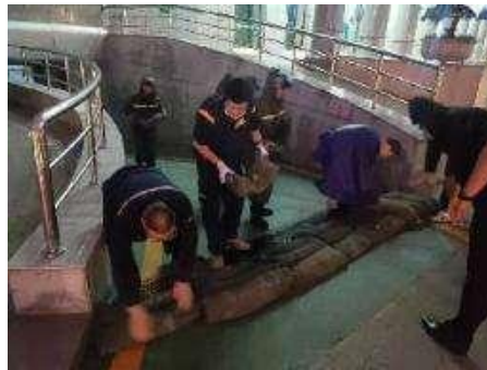
Employees of Hebei Branch deploy sandbags for flood control. (Photo by Duan Yongqiang)
