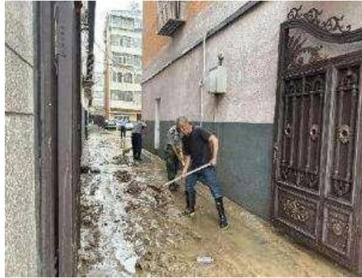
Employees of Beijing Branch help with dredging. (Photo by Wu Zheng)
