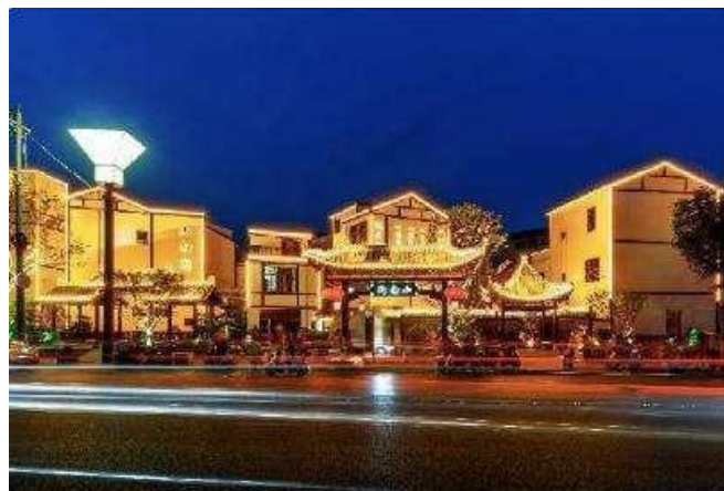
Huanggang Branch in Hubei Province supports the renovation of old town areas in
