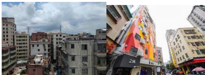
Photo: Yuanfen New Village before and after the urban renewal project
