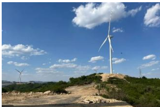
Photo: Yuedian Xinlei Wind Farm constructed with the support of Yuxian County Sub-branch in Yangquan City, Shanxi Province
