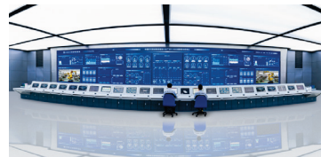
Glass fiber intelligent central control room of China Jushi
