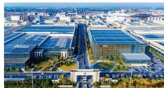
The largest intelligent manufacturing base for glass fiber in the world
