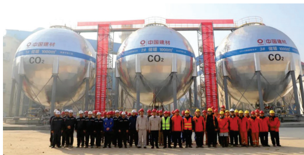
Successful launch of CUCC Qingzhou's carbon capture and purification green emission reduction demonstration project
