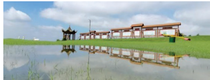
CUCC Pingyi mine ecological restoration
