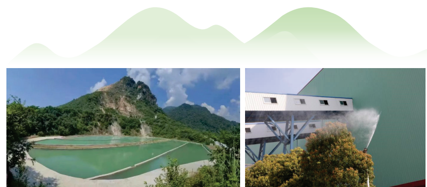
Sichuan Lisen Building Materials rainwater sewage recycling system
