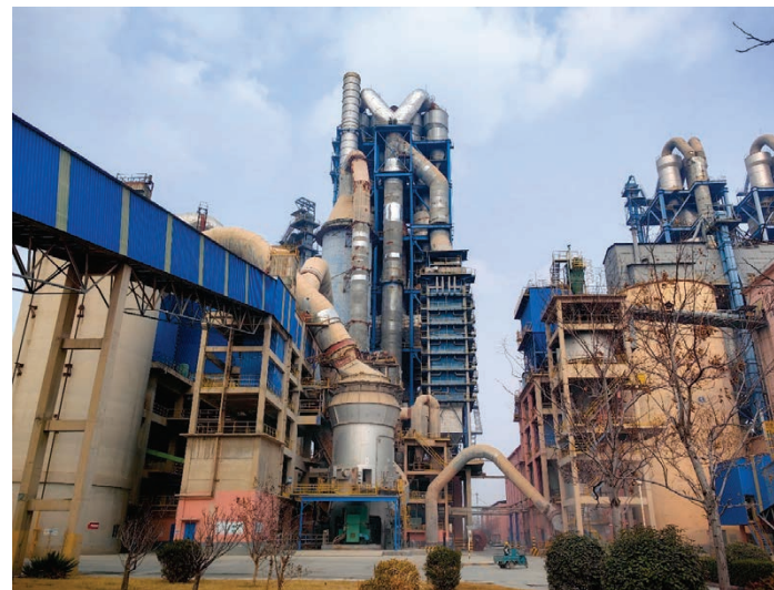
Key technology application of cement classification and separate grinding
