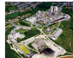
K6 oxyfuel project plant
