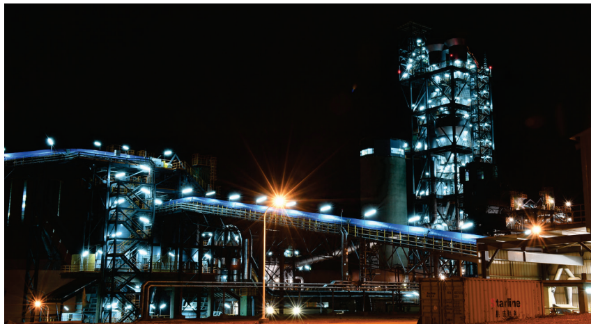
The night scene of Nigerian SOKOTO clinker cement production line
