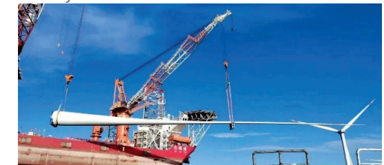
Lifting 123-meter wind turbine blades
