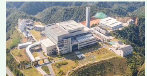
The municipal waste incineration power generation project in Ganzhou
