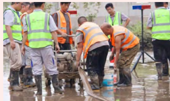
Emergency repair of the sewage pump
