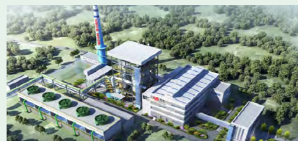
The 150MW high-efficiency supercritical surplus gas-fired power generation unit project of LY Steel
