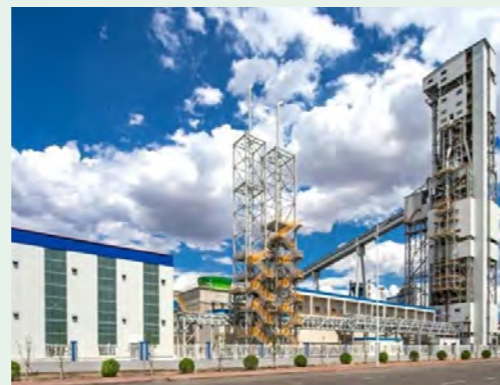
The hydrogen metallurgy project of HBIS
