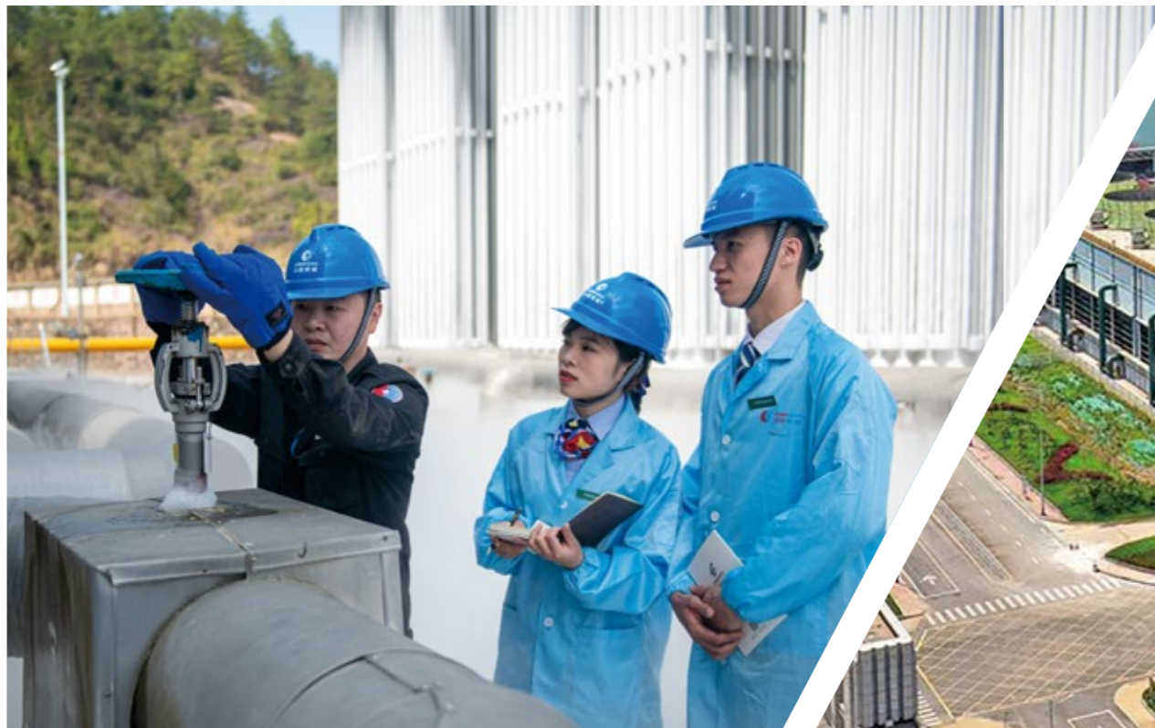
Two account managers of PSBC visited an LNG central gasification station to find out the company’s financing needs.
