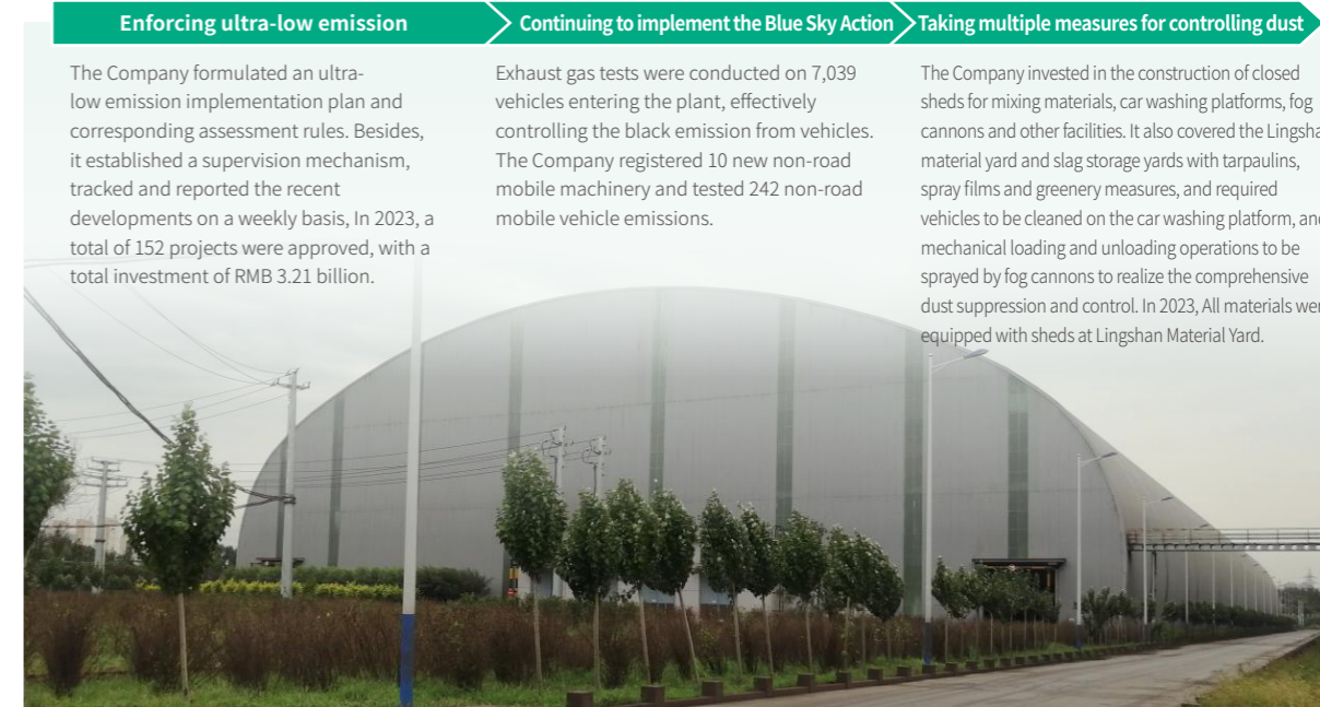
▲ Panoramic view of material shed
