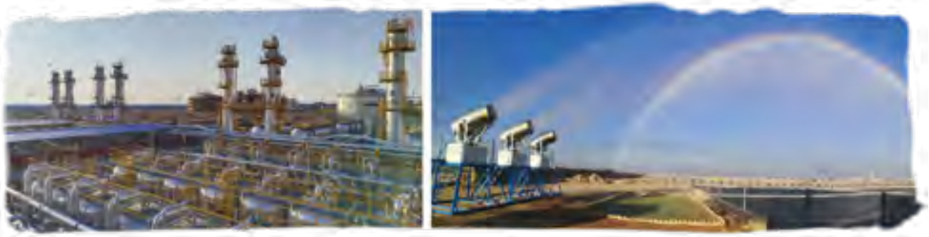
Terminal Plant Water Treatment Area of Missan Oilfield
