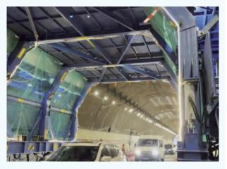
The Ningbo section in Ningbo-Taizhou-Wenzhou Expressway pioneered the development and application of intelligent and mobile maintenance cart, and achieved a breakthrough in the realisation of tunnel lining of the full cross-section and other maintenance of non-disruptive operations, reducing the impact on traffic.
