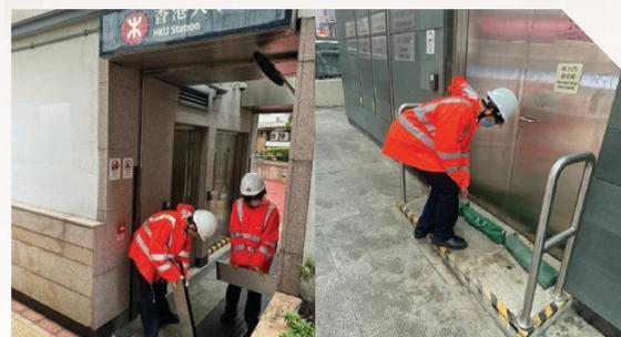
(Left) Operating colleagues installed flood boards at stations; (Right) Operating colleagues placed sandbags outside stations to prevent rainwater from entering
