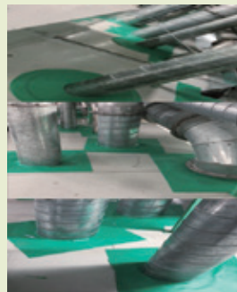
Panel holes sealing 孔洞面板封堵
