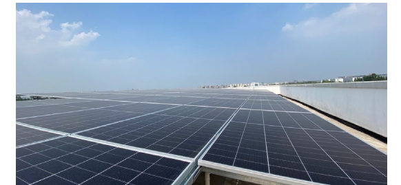
Installation of Rooftop Photovoltaics for Energy Saving and Cost Reduction
