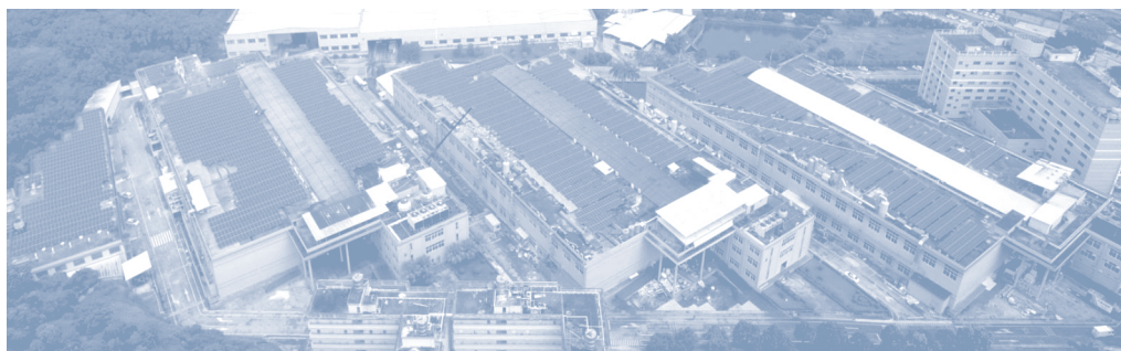
Photovoltaic clean energy project at GZXH
