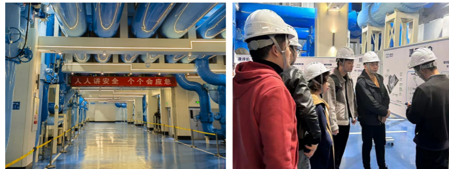
CEC Energy Conservation conducted business exchanges with CECEP City Energy Conservation
