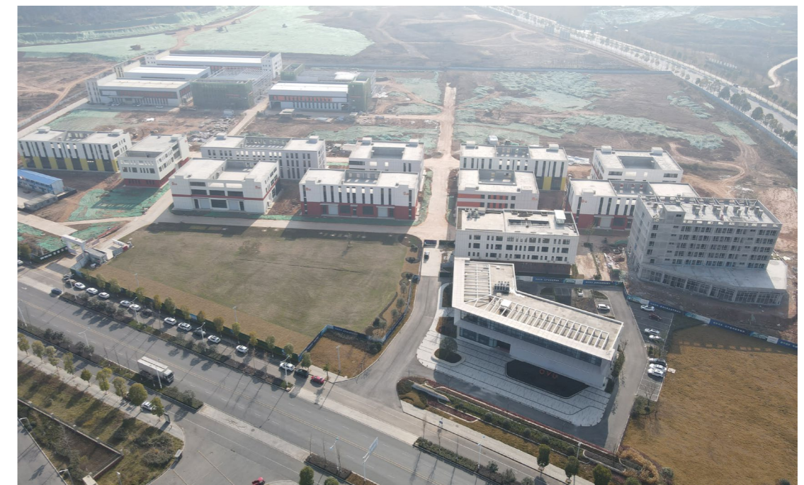
Scene of construction site
