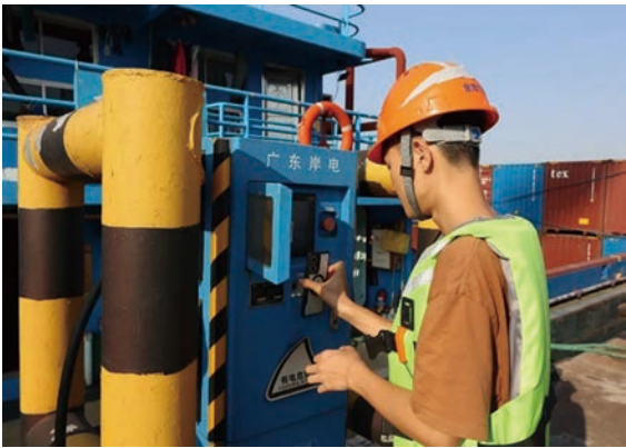
During the year, Guangzhou South China Oceangate Terminal promoted the use of shore power by vessels in port and took the lead in connecting barges at berths to shore power.
