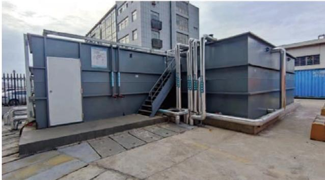
*The sewage treatment station in Lianyungang New Oriental Terminal is used to treat and purify the sewage to achieve the discharging standard or reuse.*
