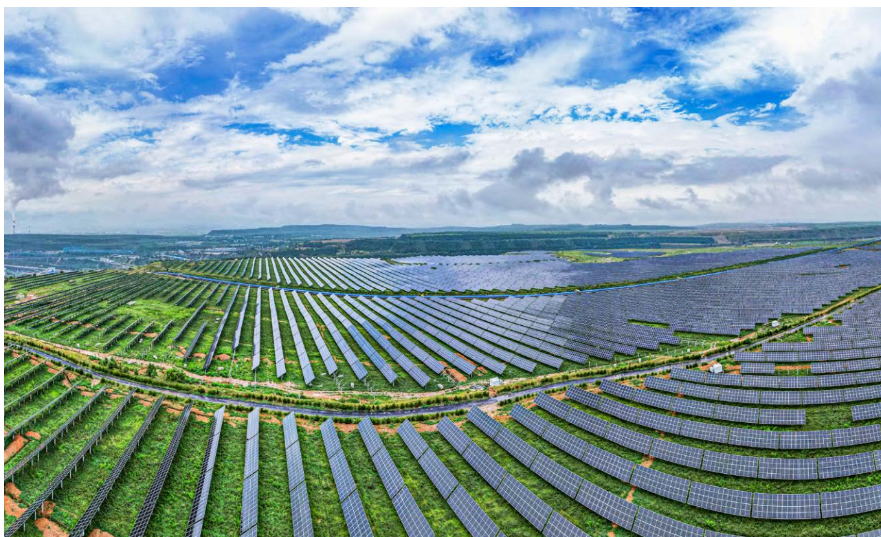
Pingshuo Group 100MW photovoltaic project
