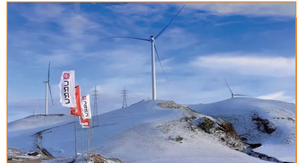
CRRC Wind Turbine Generators at the Top of Snow Mountain
