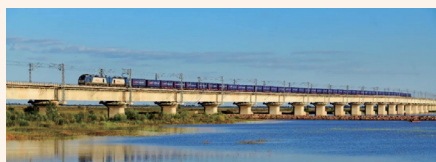
CRRC Electric Locomotives Pull China-Europe Railway Express Train through Yellow River Super Major Bridge on Datong-Xi'an Railway
