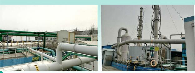
Collection and Treatment of Odorous Gases from the High-tech Park Sewage Station to Ensure No Odorous Gases Escape
