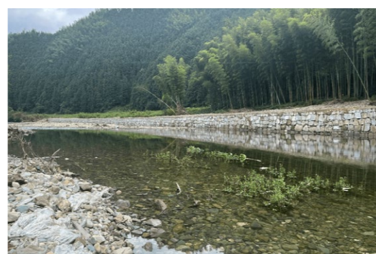
Ecological Restoration Project of the Shuaishui River Basin - after restoration
