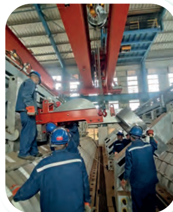
Emergency busbar installation training
