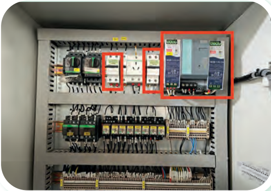
Figure 3: Shift from one-way power supply to two-way power supply for the heating quick closing valve in a thermal power plant and the control cabinet for LV valve station
