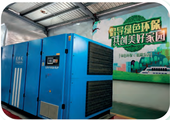
Introduction of variable frequency screw machine for gas supply isolation
