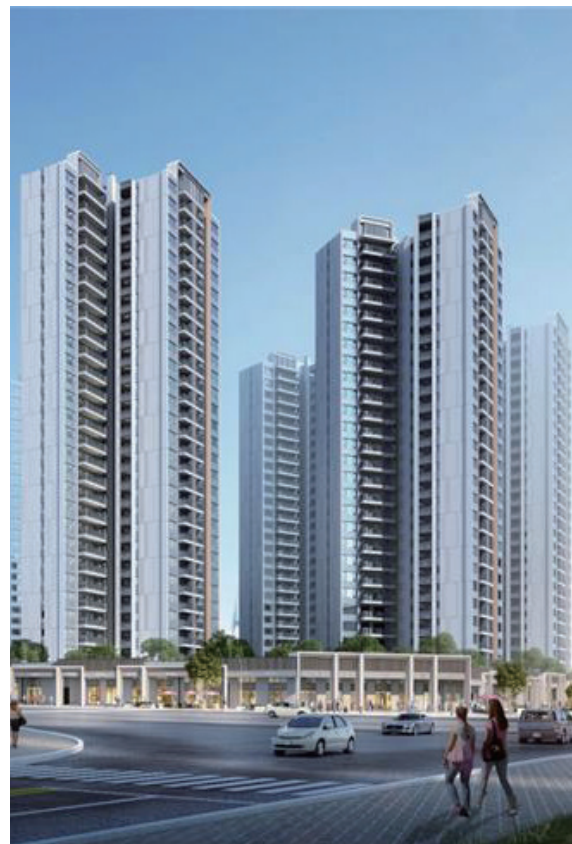
Project effect after renovation
