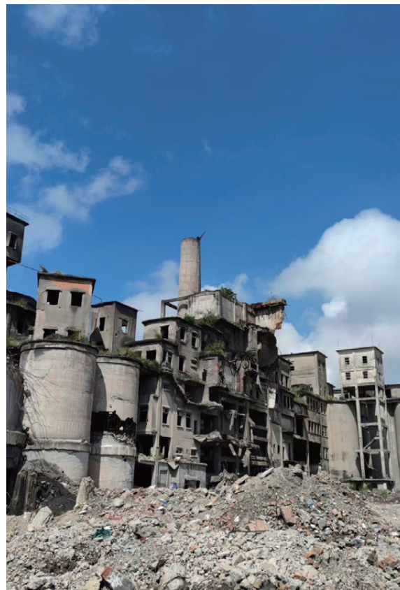
Cement Plant before renovation
