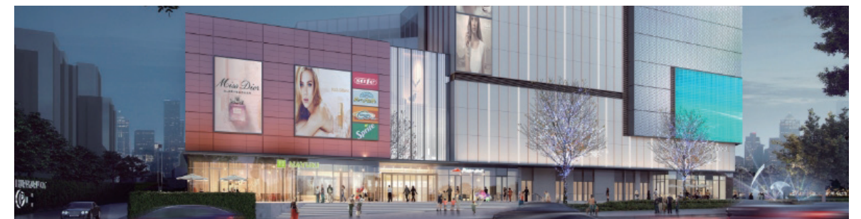
Jilin Dongshan 04 Green Building Project
