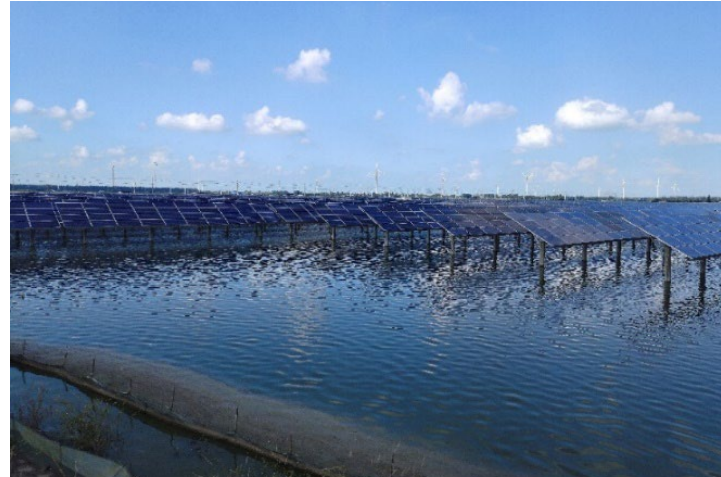
Gaoyou GCL Fishery-PV Complementary power station: Electricity Generation Above, Fish Farming Below
