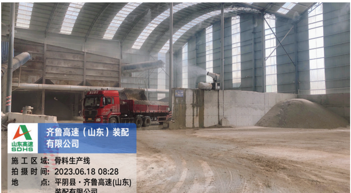
Spraying and fog cannon for dust reduction in aggregate production line workshop
