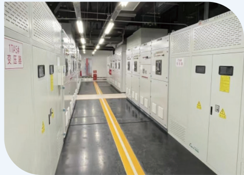
Green and low-carbon new data center construction project
