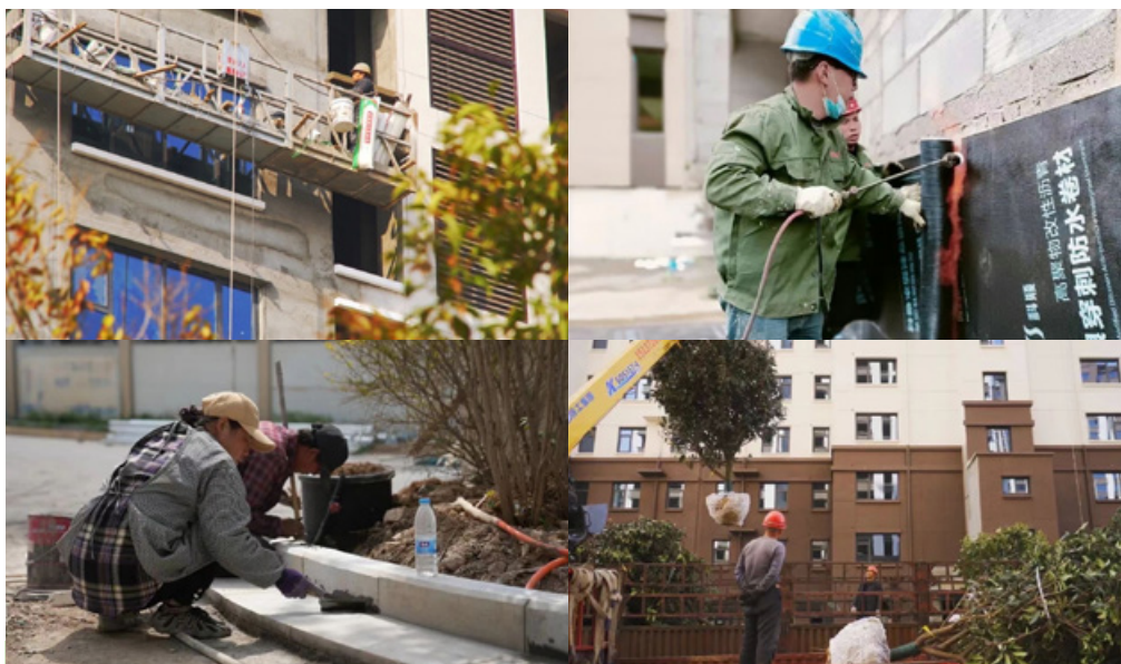
Construction sites of the Jianye project
