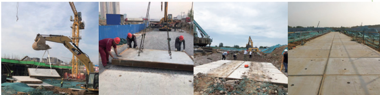
Prefabricated pavement hoisting
