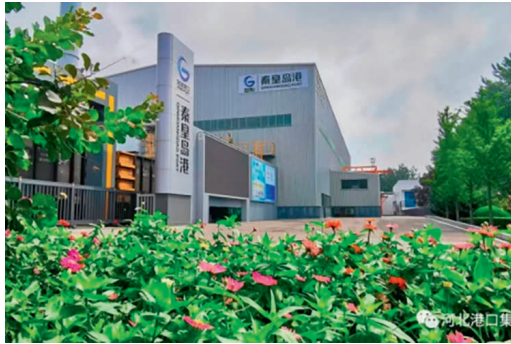
External view of the third phase of the coal turning machine room of QHD Port
