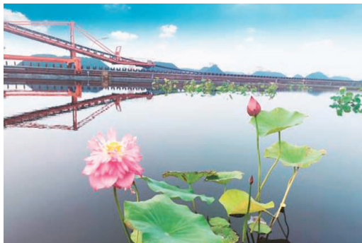
Ore yard storage sedimentation tank
