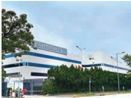
HK headquarters office cum production and broadcasting building with the outer perimeter green fence
