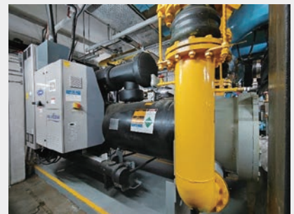
Replacement of chiller
