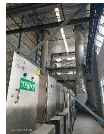
UV Photolysis and High-altitude Emission System for handling of spray paint exhaust
